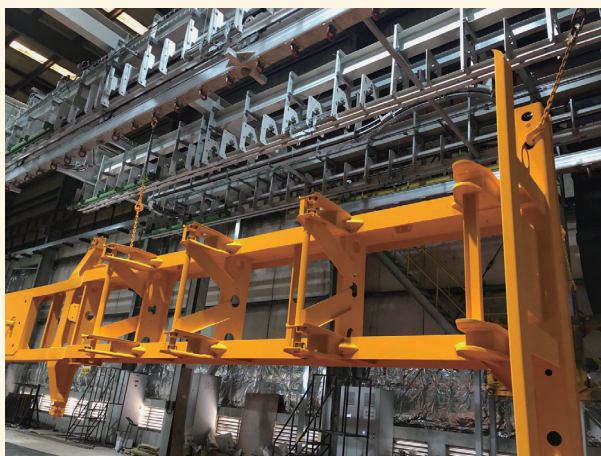
Installation of Coating System
