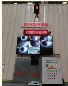
Installing Synchronous Displays on the Site
